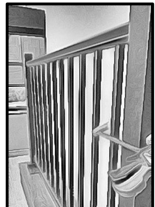
CUT PANEL AND PLACE BETWEEN POST
