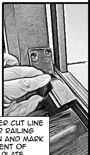
CLAMP STAIR RAIL ENDS ON POST
