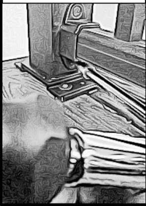
SECURE ALL RAIL ENDS WITH #14 SCREWS
