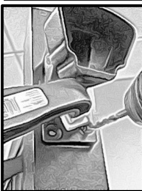
CLAMP RAIL ENDS ON POST AND PILOT HOLE AND FASTEN TO POST WITH #14
