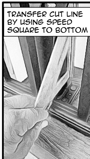
TRANSFER PENCIL LINE UTILIZING SPEED SQUARE TO TOP RAIL
