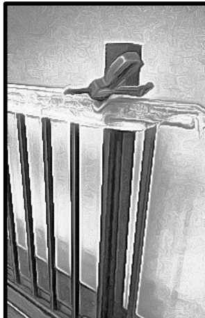
SECURE PANEL WITH QUICK GRIP CLAMP
