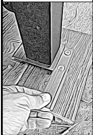
SLIDE BOSS MOUNT COVERS ONTO PLATE
