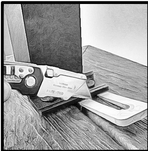
CUT EXCESS OF THE SHIM
