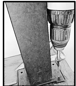
SHIM AND SCREW WITH APPROVED FASTENERS
